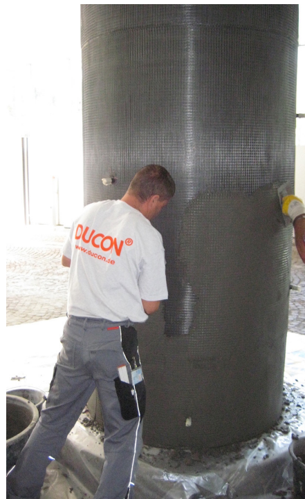
Image: Column reinforcement for explosion, impact and earthquake protection.
