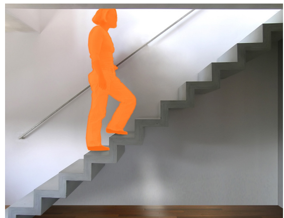
Image: cantilever folding staircase d=80mm = thinnest concrete stairs
