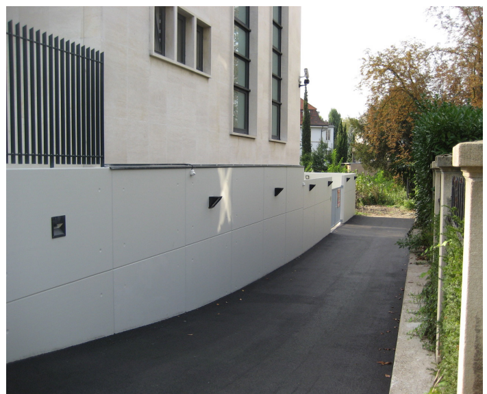
e.g. Protective façade Consulate General
