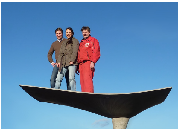
Image: "Parapluie" d= 25 – 30mm = thinnest roof shell
