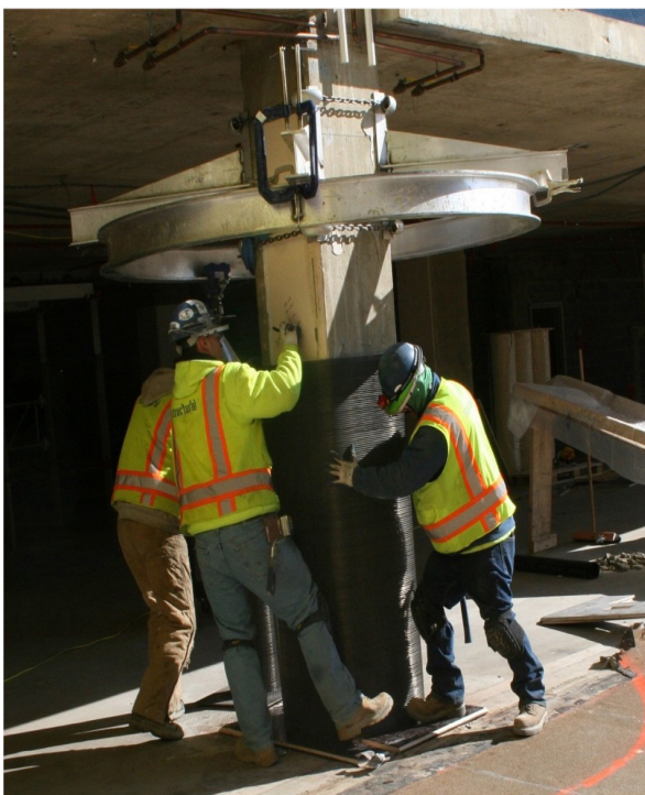
Image: Column reinforcement for explosion, impact and earthquake protection.
