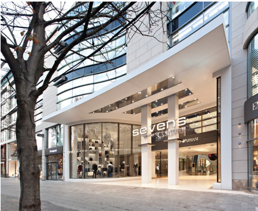
Fig. 17: Finished Entrance of "Sevens" (pict. RKW architects), all elements 50 – 70 mm thin
