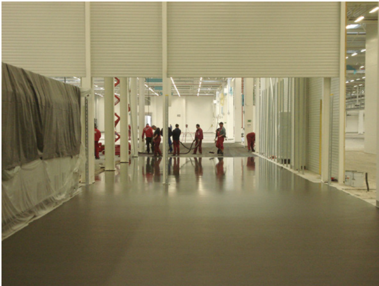
Fig. 27: DUCON® joint-less ( d = 30\text{ mm} , 1.2")
