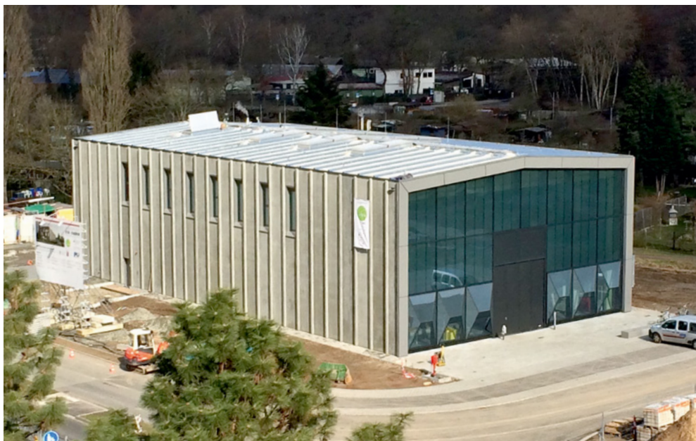
Fig. 32: Installed façade (h=10,6 m, 35 ft / l=42 m, 140 ft)
