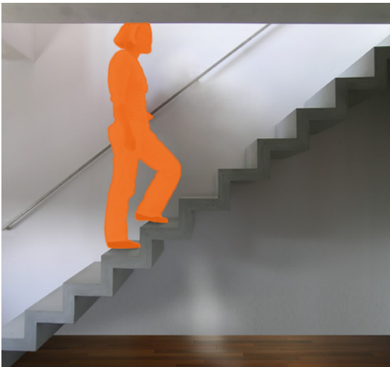
Fig. 7: Free-span folded stair (d = 80mm, 3.2")
