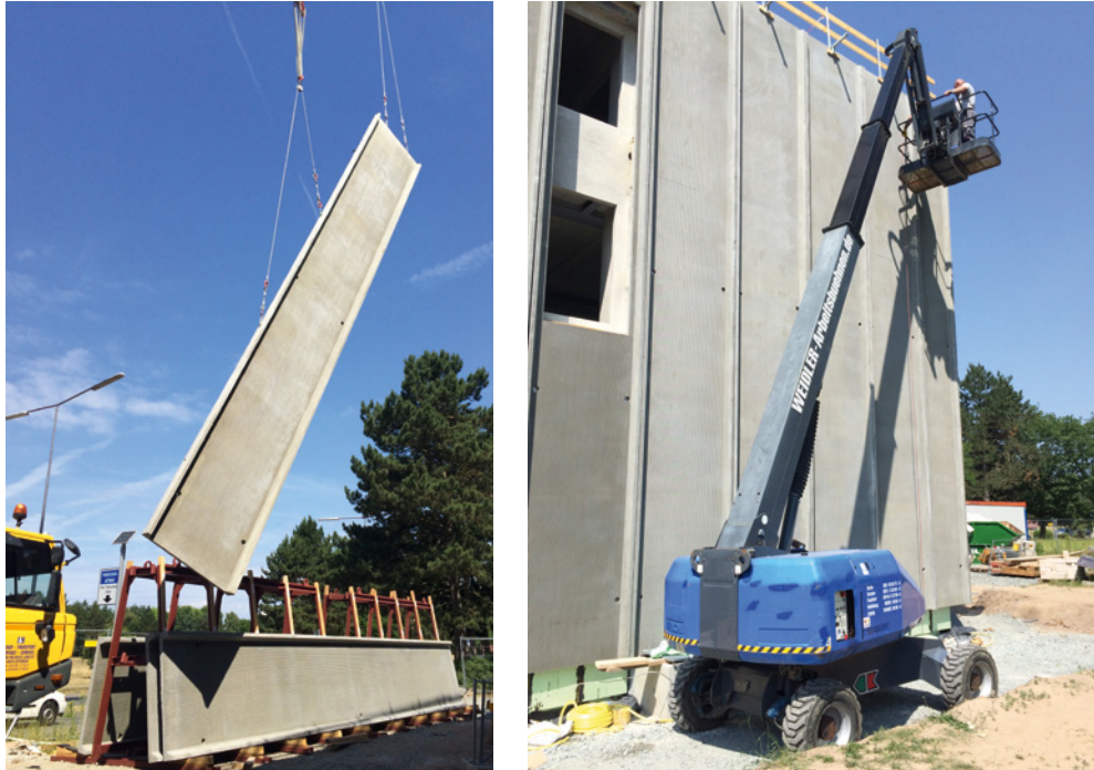
Fig. 31: Site-installation of façade and roof panels
