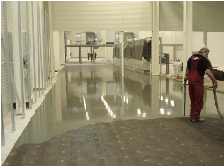
Fig. 26: DUCON-slurry infiltration into MicroMats®
