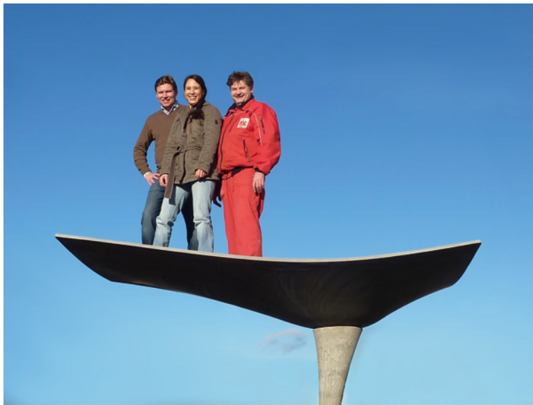
Fig. 4: “Parapluie” – ultra-thin roof panel, (d=30 mm, 1.2”)
