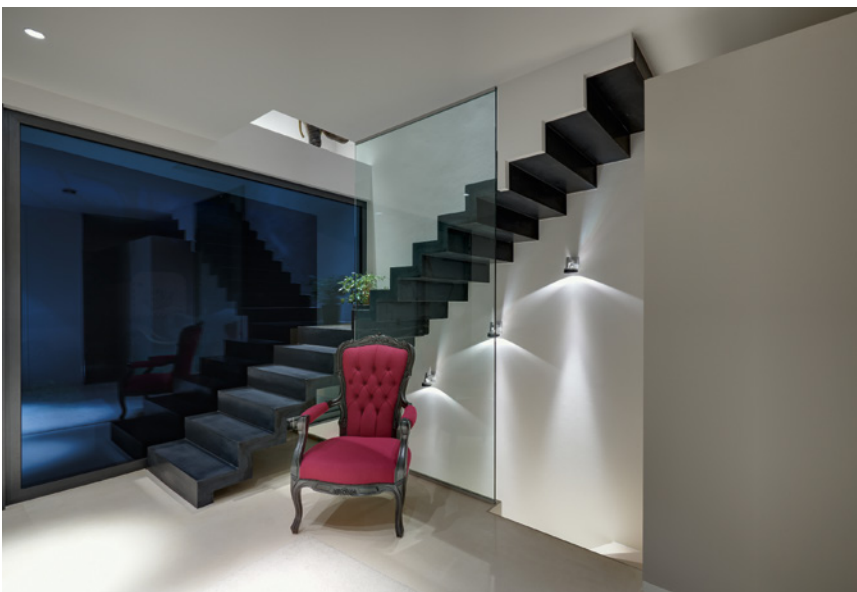
Fig. 9: Black folded stair system (d = 95 mm, 3.7")
