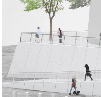
Fig. 19: Façade panels (d = 30 mm, 1.2")
