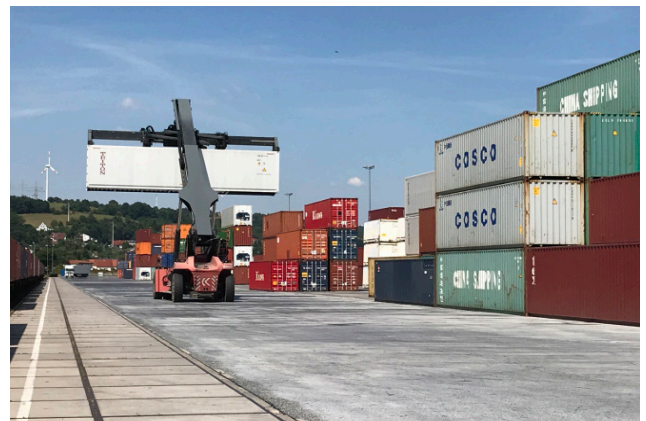
Figure: Heavily loaded base course and sealing layer (6,000 m 2 container storage area, t = 55 mm)
