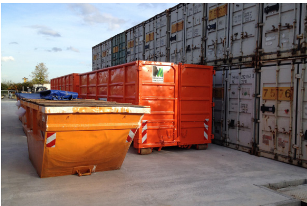
Figure: Heavily loaded base course and sealing layer (6,000 m 2 container storage area, t = 55 mm)
