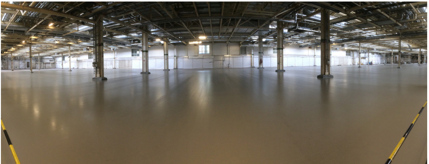
Figure: WHG sealing layer, d=55mm, 15.500m 2 seamless, automotive industry
