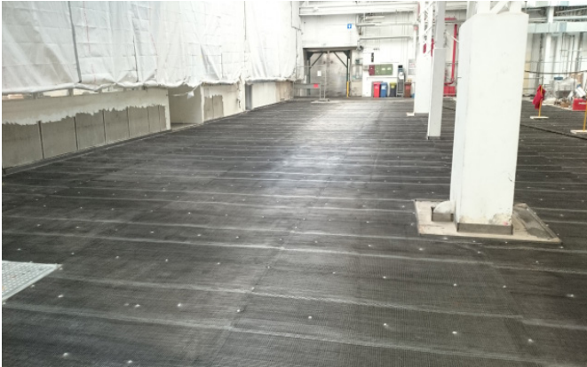
Figure: Laying of the micro-reinforcement MicroMat®
