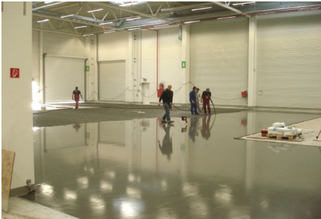
Figure: Concreting with DUCON1 concrete
