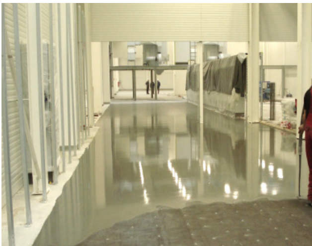
Figure: Construction of a ceiling reinforcement (t = 60 mm)
