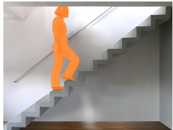
Figure: Self-supporting folding staircase, t=80mm
