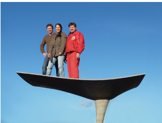
Figure: "Parapluie" d= 25-30 mm = thinnest roof shell
